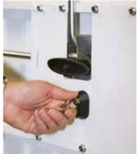
The reinforced locking barrel includes a key for locking and unlocking from the **inside** of your garage. The door is fully operational from both inside and outside of your garage.
