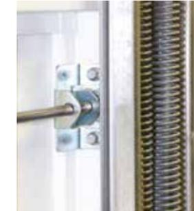
3-point solid bar locking fully supported across the width of the door.
